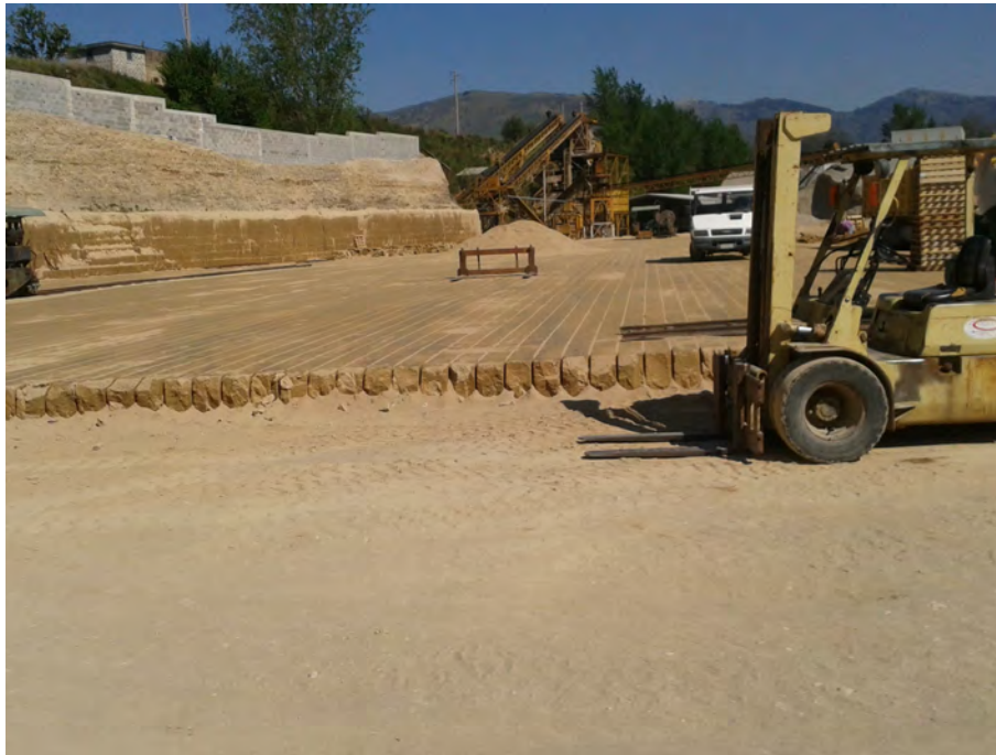
Figure 2 – LS quarry (see Fig. 1), Comiziano, some 26 km, NE of Naples.
